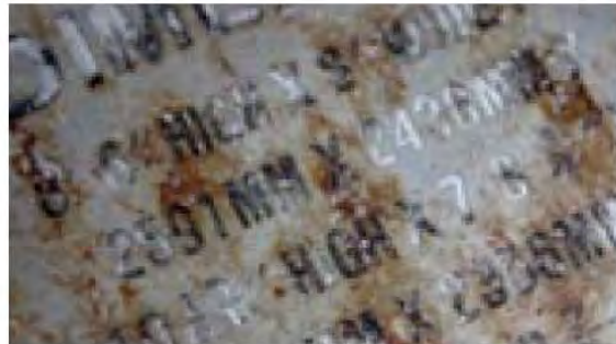
Road Salt Corrosion Damage
